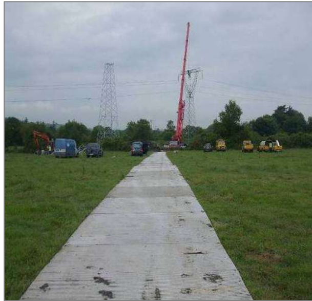
Figure 7: Temporary Aluminium Panel Tracks
