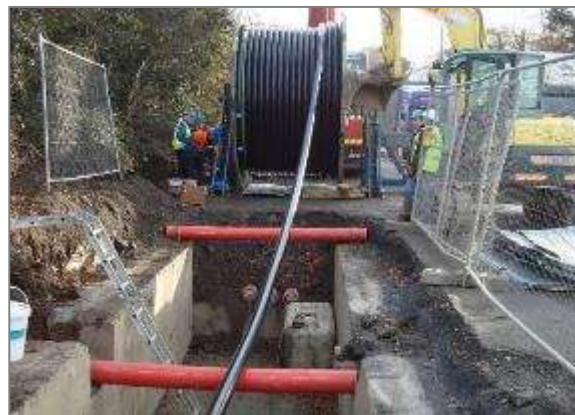
Figure 5: HV cable pulling procedure (Typical drum set-up)
